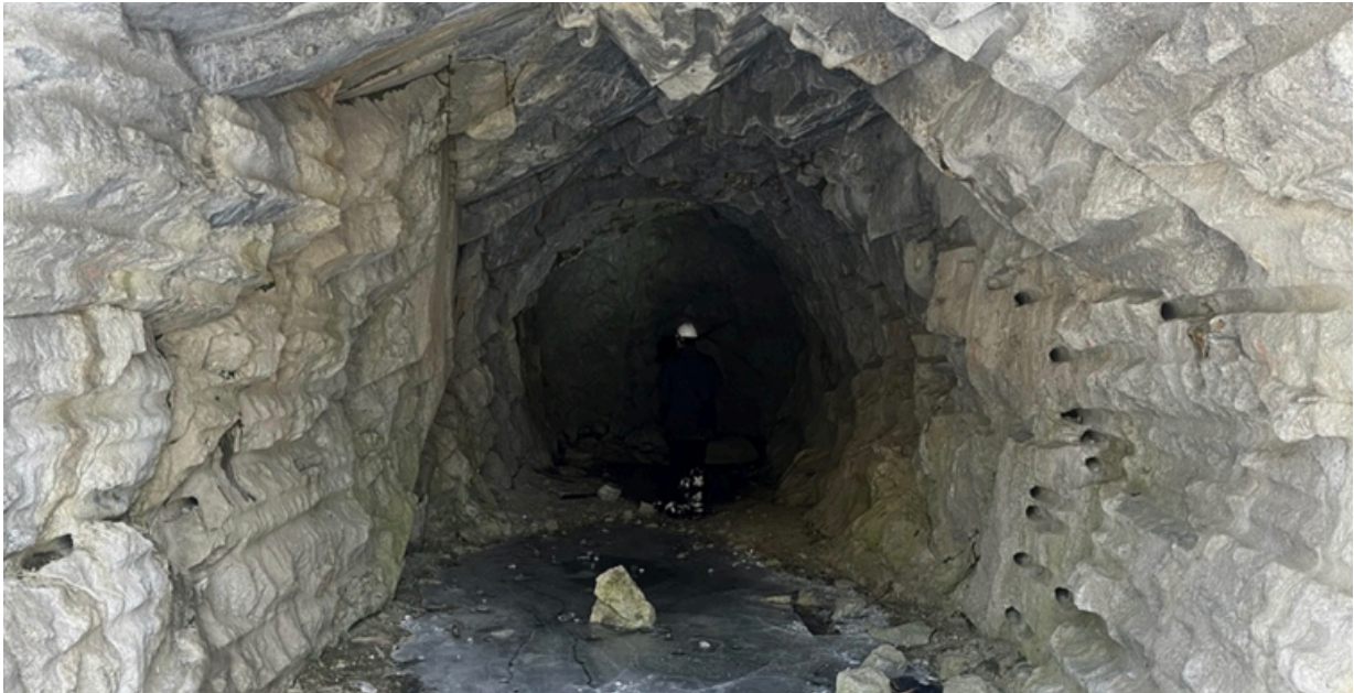
Figure 1: The World's first Hypersonic-Bored Tunnel. Project REAM
